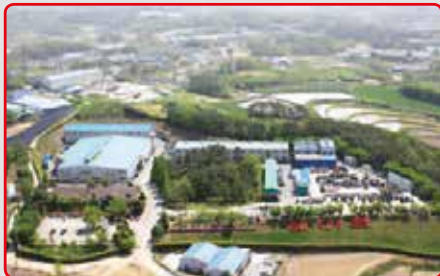
Cargotech Korea Co., Ltd. factory view
